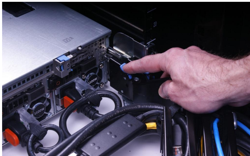
Figure 7. Disconnecting the CMA attachment housings
